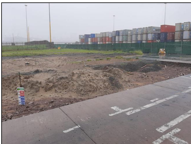
3) Test piling completed on site. - November 2020
