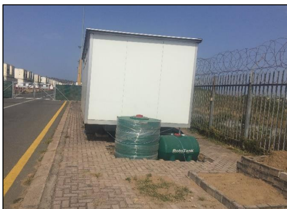
16) Installation of wastewater tanks at the shower room – November 2020
