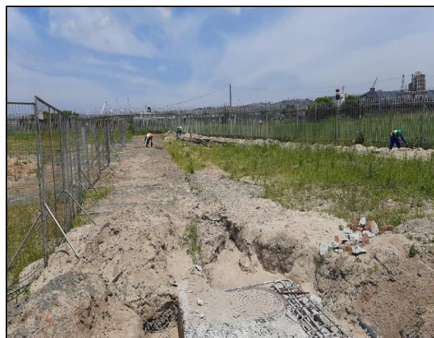
4) Temporary fencing and the removal of cables on site. – December 2020
