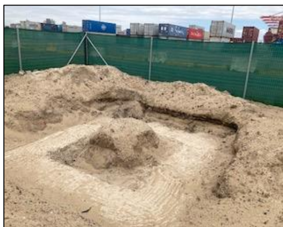
5) Preparation for construction of concrete platform on site. – January 2021
