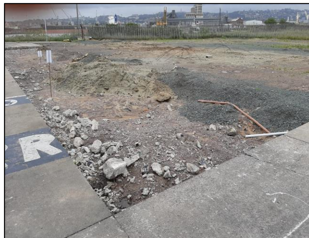
2) Test piling completed on site –October 2020.
