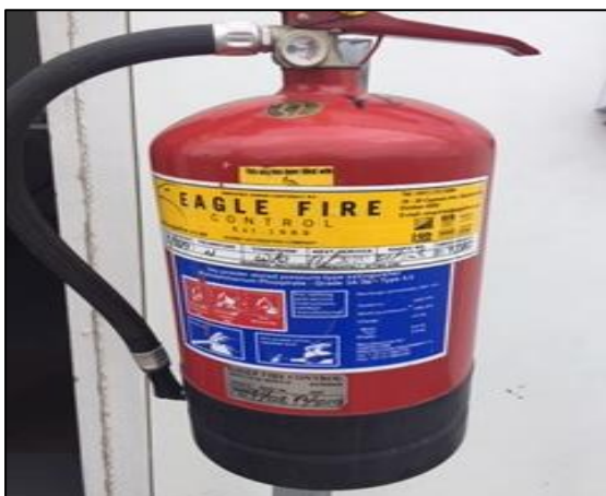
10) Provision of fire extinguishers on site – September 2020
