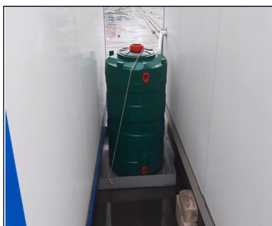
17) Waste water tank used on site. – November 2020
