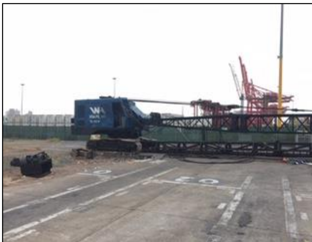
1) Plant on site ready for piling. –September 2020
