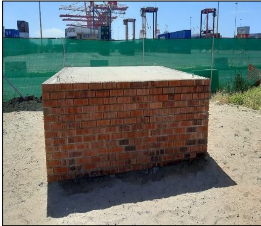
7) Construction of concrete platform on site. - February 2021
