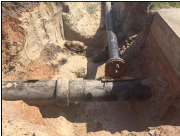
1) Asbestos pipe to be removed from site –March 2020
