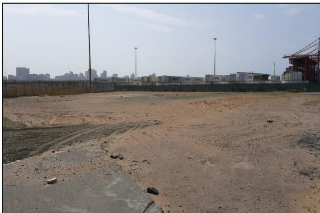
3) The construction site is clearly demarcated- August 2020
