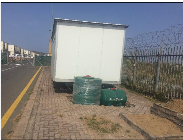
8) Installation of wastewater tanks at the shower room – August 2020
